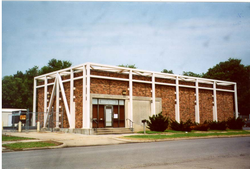
Figure 18. Seismic retrofit structural steel frame around telephone company building in New Madrid
